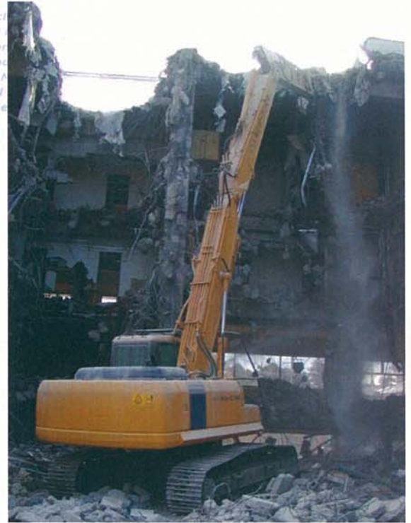
Demolition work in progress
